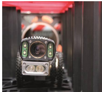
Inspection with camera
